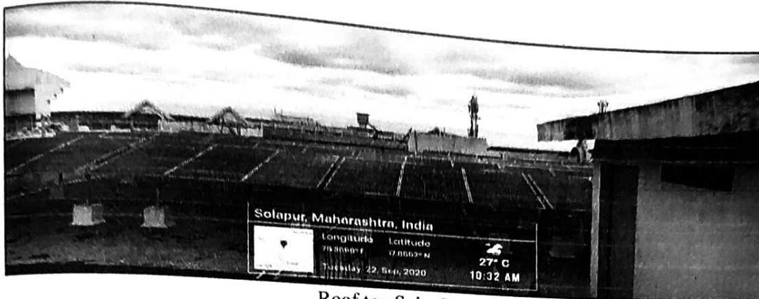
Roof top Solar PV
