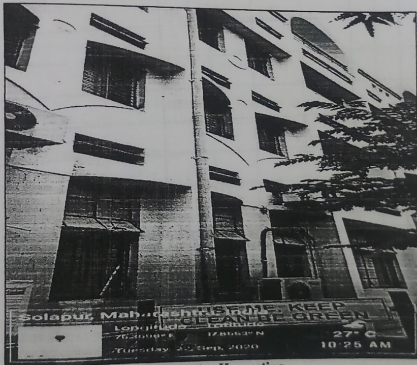
Rain water Harvesting
